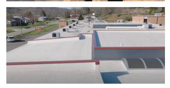
Once the insulation installation was complete, Duro-Tuff membrane was induction welded to the surface, creating a watertight finish over the entire 66,000-square-foot roof. Finally, custom Duro-Last components including gutters, downspouts, 2-Piece Snap-On Compression, termination bars and flat copings completed the installation. Additional features such as roof drains, ROOF-TRAK III walkway pads and Knucklehead extensions enhanced functionality and safety.
