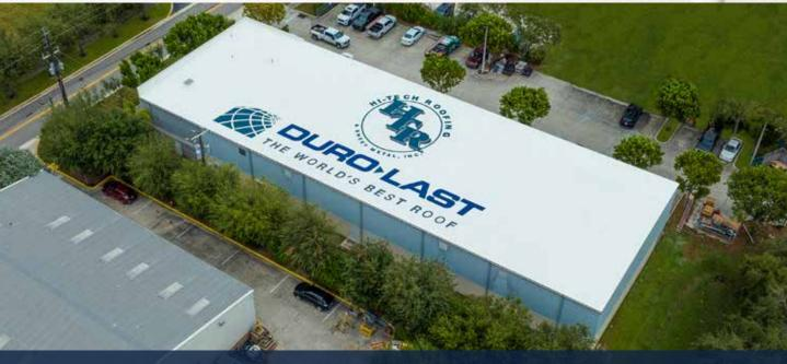
Location: Lake Worth Beach, Florida Square Feet: 16,200 Products: Custom-fabricated Duro-Last 50 mil white membrane; Duro-Guard® EPS Flute Fill insulation; Duro-Guard 2.5" ISO insulation; Duro-Bond® induction plates; fascia; custom rooftop logos
