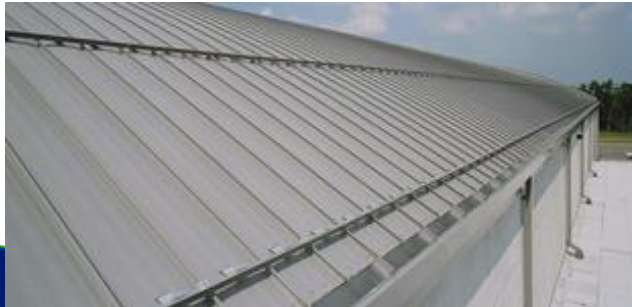
Mechanically field-seamed, high strength structural
