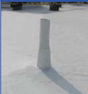
Duro-Last's stacks are also custom prefabricated under ideal factory-controlled conditions, from 1" diameter to any required size. Factory prefabrication reduces field labor costs and leaks common to site-created flashings.
