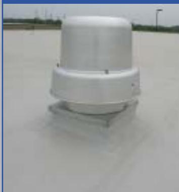
One-piece custom prefabricated curb flashings are made to the exact size of the units on your roof. Other systems require hand cutting and the fitting of as many as eight pieces of material for each curb. The result - less labor and a more efficient installation.
