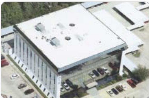
Complete roofing system
