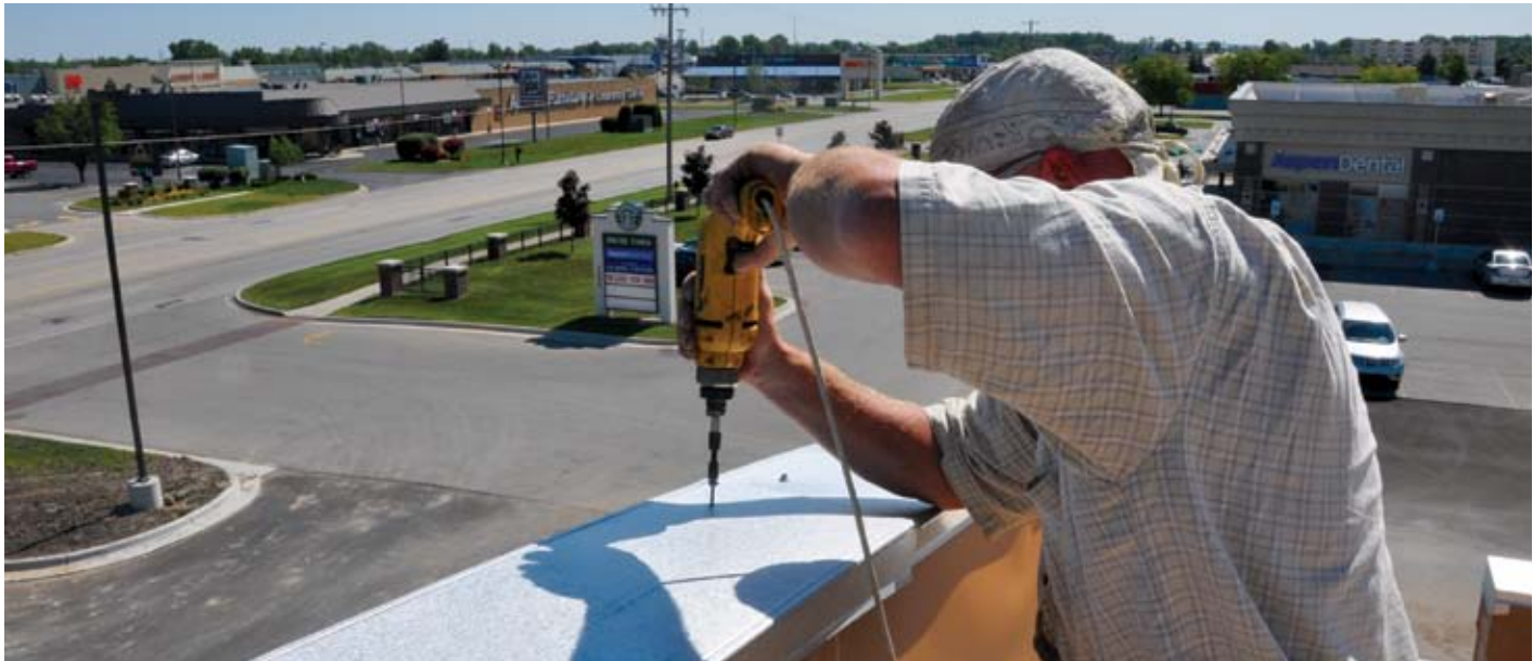
COURTESY DURO-LAST ROOFING, INC.:
