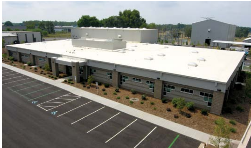
COURTESY DURO-LAST ROOFING, INC.
