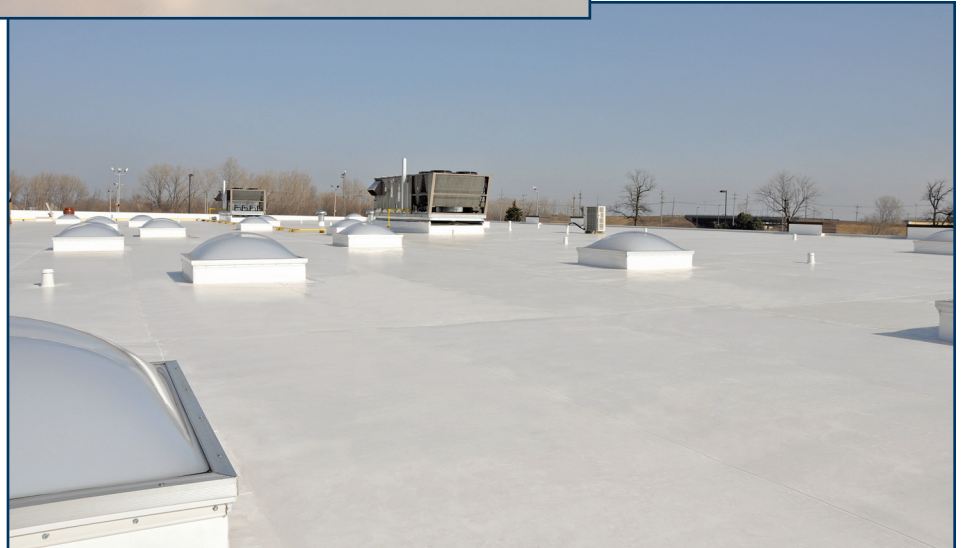
Figure 3 – Custom prefabricated curb flashings.
